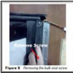
Figure 8 Removing the bulb seal screw
