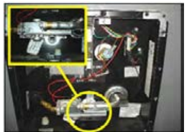
Fig 1: Water heater drain plug
